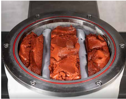
Streamer in heat exchanger
